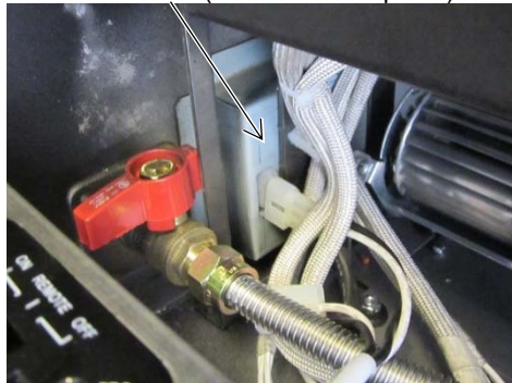
Junction Box (from inside fireplace)
