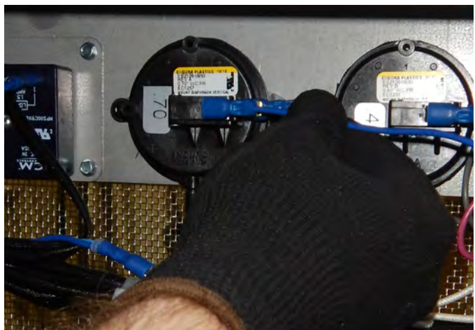
Figure 116. Disconnect blue wire.
