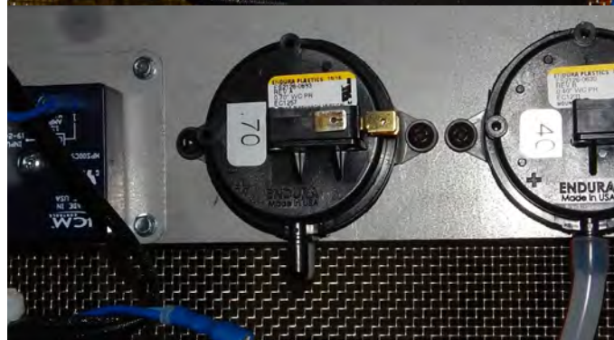
Figure 117. Disconnect grey wire.
