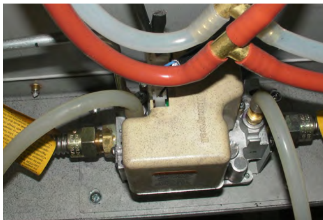
Figure 51a. Pressure Testing (viewed from rear of appliance)
