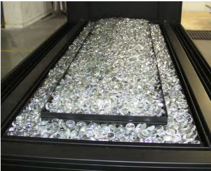
Figure 60. Firestones in upper and lower trays.
