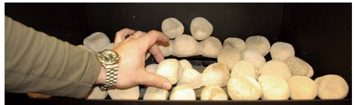
Figure 23.n Place the first Top faux Rock.
