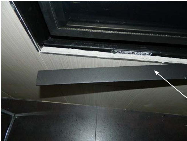
Figure 101: Top View - Sliding trim into place
