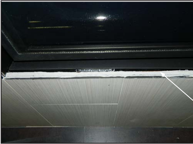
Figure 100: Top View - exposed non combustible materials
