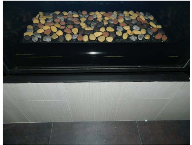
Figure 102: Completed Trim install
