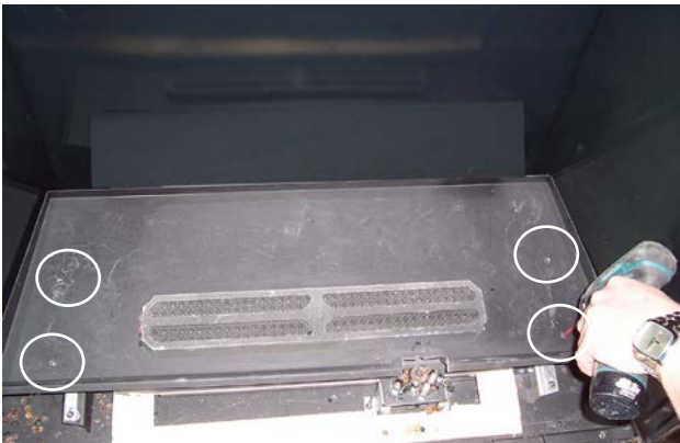
Figure 64: Burner Screw Locations
