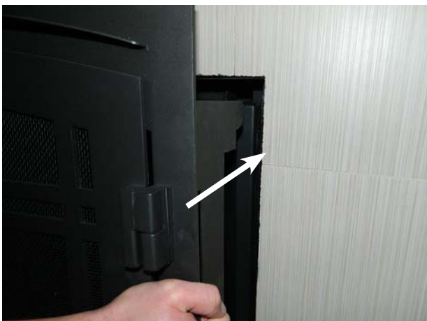
Figure 98: Line up Tabs with slot on Unit
