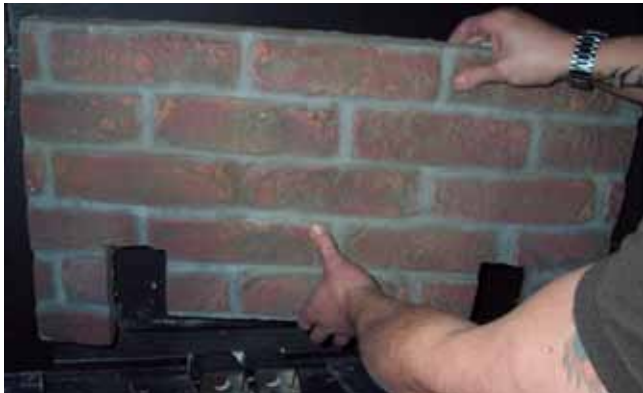
Figure 77: Lower Back Brick Panel
