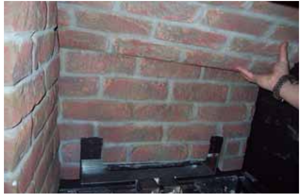
Figure 79: Upper Back Brick Panel
