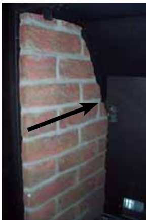
Figure 78: Left Brick Panel
