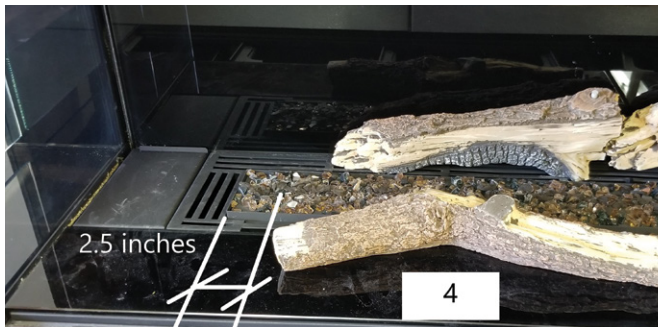
Log 4 to edge of burner
