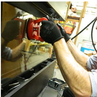
Handle glass with supplied vacuum clamps
