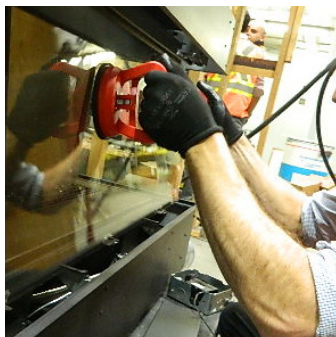
Handle glass with supplied vacuum clamps
