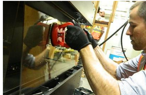
Handle front panel with supplied vacuum clamps
